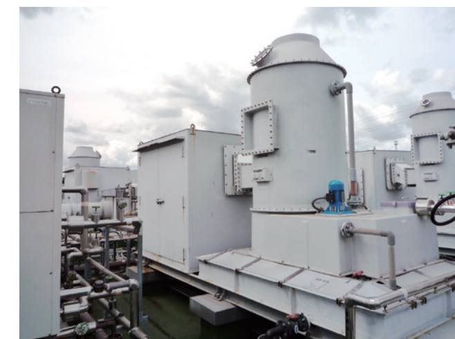
Exhaust cleaning towers at the R&D Center
